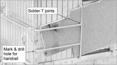
these joints using 60/40 electrical solder as this gives a stronger joint than using 145° solder. Use plenty of flux and make sure the solder runs all around the joint. You will have to mark and drill a hole in the corner strapping for the bottom horizontal handrail. Also note that some vans had extra horizontal handrails fitted by the LNER (see scale drawing) and if fitting these mark and drill extra holes.
